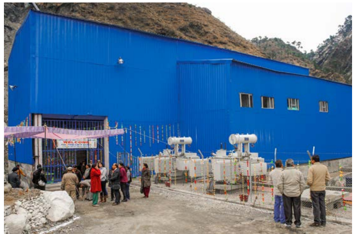
Opening of the Ayush hydro-electric facility | Himachal Pradesh, India
