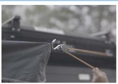
8. Hook the tensioner rope onto the eyelet
