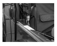
**Step 4:** Take a mounting bracket and place it in position on the tub centered around the mark you made in Step 3.
