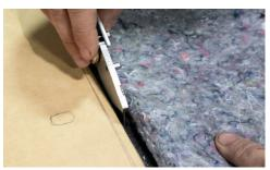
• Using a razorblade, cut a slot between the marks in the carpet.
