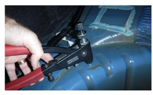
**Step 7:** Install the provided 1/4"-20 Rivet Nuts in the 5 holes.
