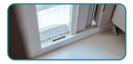
Position both bottoms of side panels into bottom of window channel track.
