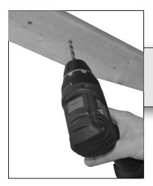
Using a 3/16" bit, drill pilot holes in all four marked mounted hole locations.
