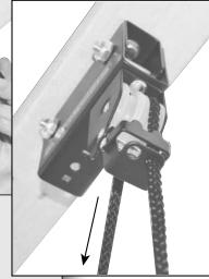
Pull the free end of the Pulley Rope down to the floor.
