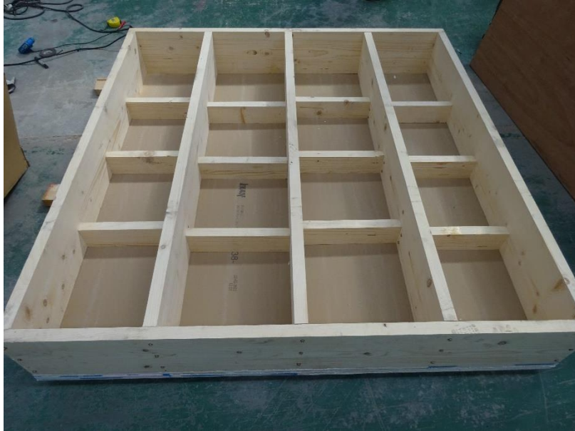
Photo No. 5 Ceiling Assembly Being Constructed
