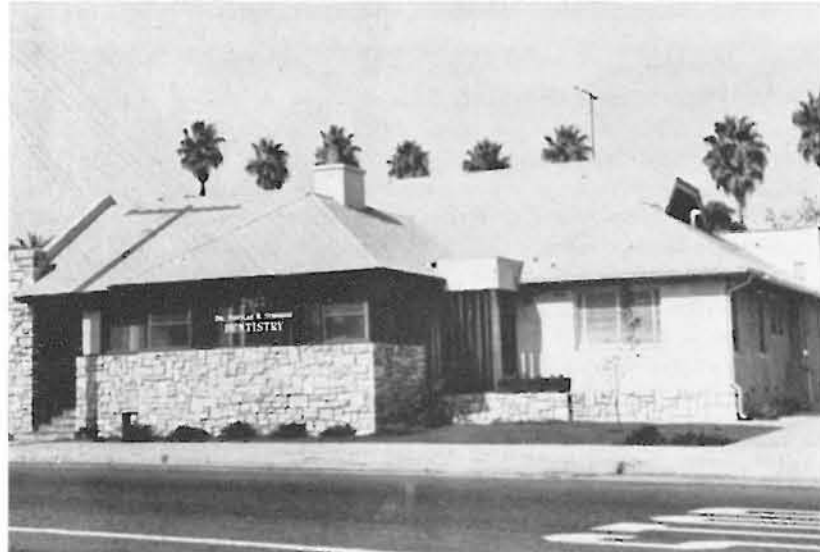
After. House stuccoed to conform with new office, and old screens replaced with modern aluminum tension screens. Rock trim is Arizona Mint stone, a pale orchid and green natural rock.
