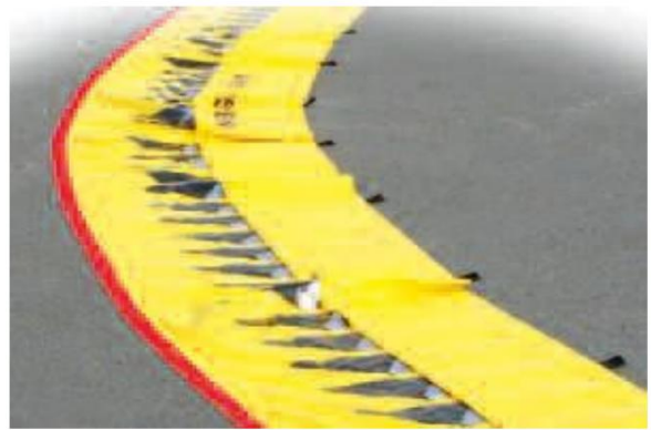
2 – Round your barrier to the desired curve.
