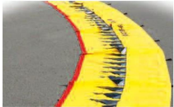
2 – Round off to the desired curve, ensuring that the back of the barrier is not stretched.
