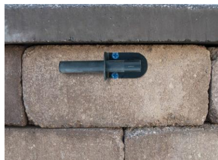
Figure 6.5 – Fasten down the bracket
