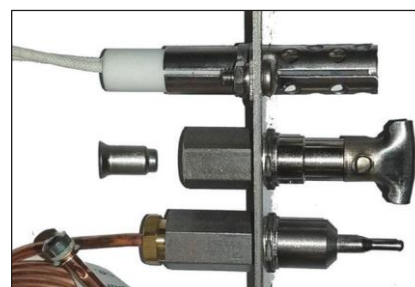
Figure 9.3 – Cleaning pilot orifice
