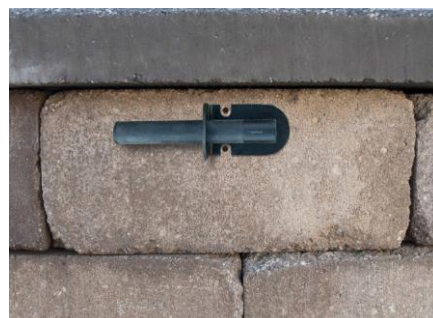
Figure 6.4 – Dry fit the bracket
