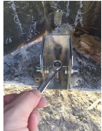
Place anchor and tighten
