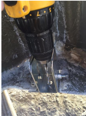
Drill through ground
