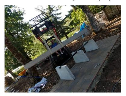
To place the table top, center over the legs and lower slowly. Place table with packaging wrap in place to avoid damaging the concrete. Two men should make manual adjustments while the table is supported by lifting equipment to align the bolt holes in the steel runners under the slab with the threads on the underside of table top.
