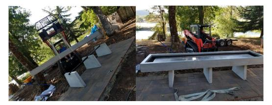
Lift concrete table with 12' or 14' foot straps placed over the packaging padding wrapped on the four corners. Use a shackle or lifting hook and rig straps as shown below.
