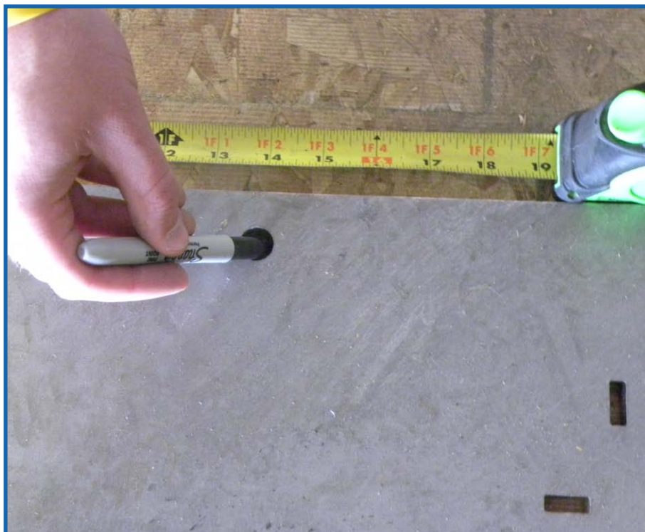
MARK THE FOUR MOUNTING HOLES
