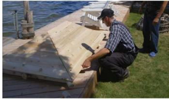
Install the bottom roof boards in the same manner.
