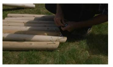
To make installation easier, pre place 3" (76mm) screws into the ends of the roof supports.
