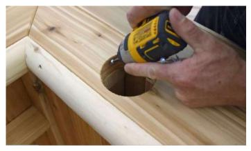
If the roof option is chosen, secure the bar top to the base through the post holes.
