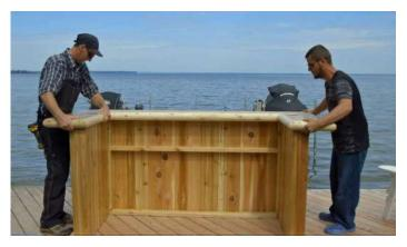
Place the bar top onto the assembled bottom base.
