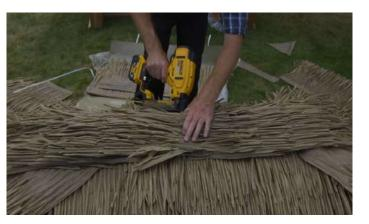
Overlap the 2 cut pieces back to back then secure into place with staples.
