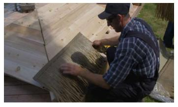
Place the thatch onto the roof with the synthetic palm leaves hanging over the bottom as in picture.
