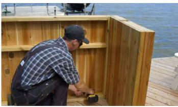
Holding the walls flush together, secure them using the provided 2 ½" (64mm) screws from the inside of the front wall into the side wall.
