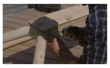
Position one of the shorter supports flush to the side and top of the side of the roof cap and secure with 3" (76mm) screws.
