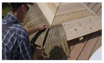
Use the cut off piece to start the first row on the short side. Cut the excess off the corner in the same manner.
