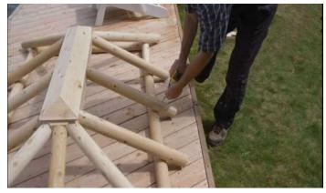
Screw the bottoms of the roof supports to the roof frame using 3" (76mm) screws.
