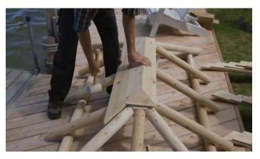
Starting on one of the sides, insert the shortest board up tight to the roof cap.
