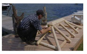
Center 1 roof support on the end and secure as in the previous step.
