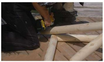
Screw the corners of the roof supports to the roof frame using 3" (76mm) screws.
