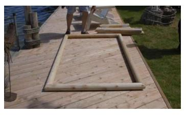
Lay the roof frame on a clean flat surface.
