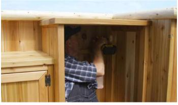
Repeat the process by fastening inside the mini fridge compartment to the tiki bar base using 2 ½" (64mm) screws.
