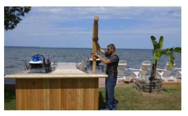
Insert the bar posts into the holes on the top of the tiki bar.
