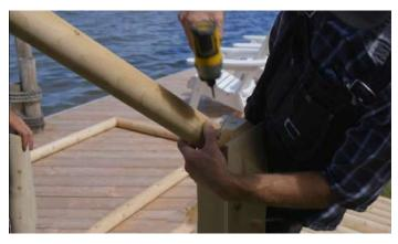
With assistance from a helper, hold the corner roof support flush to the corner of the roof cap assembly. Secure the post to the assembly with 3" (76mm) screws.
