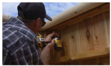
Secure the base to the bar top using the provided 2  $\frac{1}{2}$ " (64mm) screws from the inside of the front wall up into the bar top.
