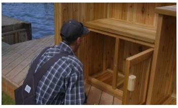
Secure the frame on the inside of the bar cabinet to the tiki bar base using 2  $\frac{1}{2}$ " (64mm) screws.
