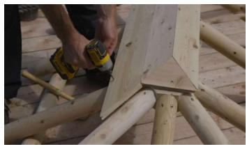
Secure the roof boards into the roof supports with the provided 2" (51mm) screws.
