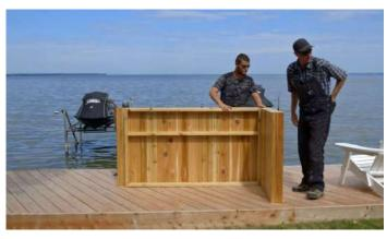
Slide one of the side wall pieces flush into the front wall.
