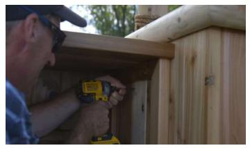
Secure the bar posts from the inside of the base using the provided 3" (76mm) wood screws.
