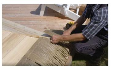
When you get to the end of the roof, cut off the excess thatch with a utility knife.
