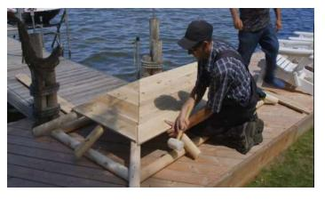
Continue adding the roof boards working around the roof assembly.
