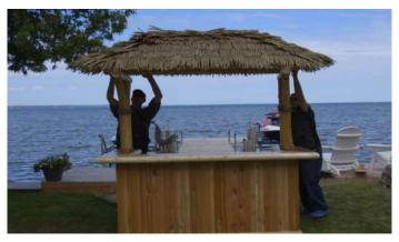
With a helper, place the roof up onto the bar posts.
