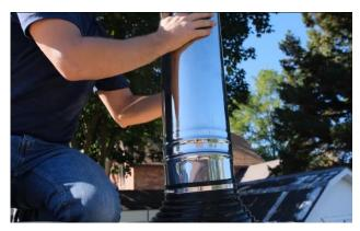
Place the 2<sup>nd</sup> insulated chimney piece over the first.
