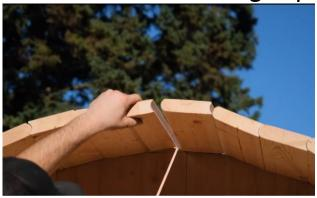
In your sauna package you will find a spacer stave that is square on both sides that is only required If there happens to be a "gap" after installing all the staves like in the picture on the left.
