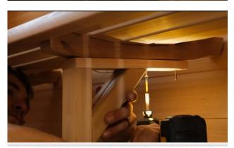
Place the bench support bracket under the seat supports and secure with 3 – 1 ½" (38mm) screws.
