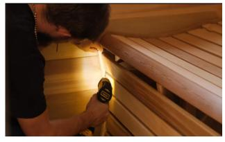
Secure the front enclosure the wall and the bench supports using 1 ½" (38mm) screws.
