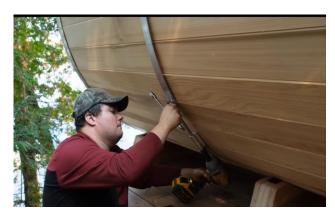
Feed another band over and under the sauna and secure it with a rod and nut.
