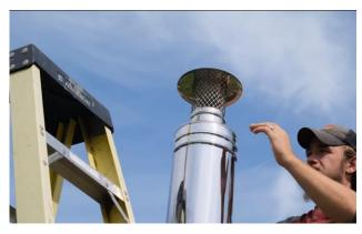
Install the cap on the top of the assembled chimney.
