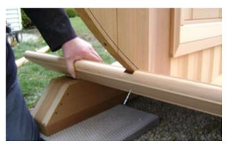
When installing the staves, tap tightly together while leaving as much of a gap as possible between stave and wall using the pencil line as a guide as in picture.
