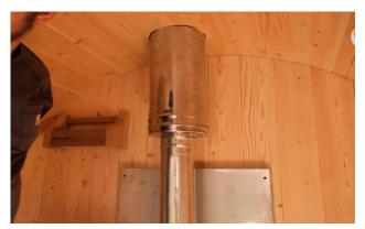
Place the first thick insulated chimney pipe on top of the first pipe and put it through the hole in the roof.
