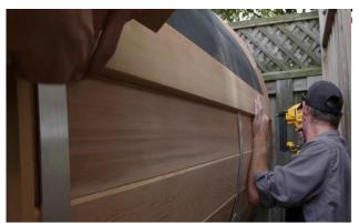
Line up your first piece of bevel siding at  $48 \frac{1}{2}$ " (123 cm) from the ground.
