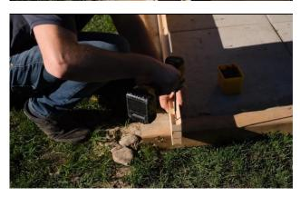
Now screw the other side of the top stave back to the other half top stave and it should now make a "V" shape when wedged with the last stave on the sauna.
