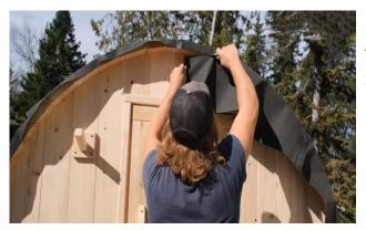
Using a utility knife, cut off the excess rubber flush to the edge of the staves on the front and back of the sauna.
