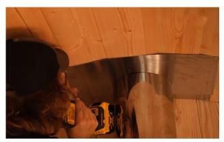
Install the 2 halves of the thin metal sheeting around the chimney on the inside to cover the hole.
