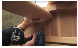
Secure with 2 ½" (64mm) screws from the underneath.
