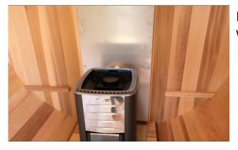
Ensure the rear wall heat shield is level and secure with  $6 - 1 \frac{1}{2}$ " (38mm) screws through the drilled holes.
