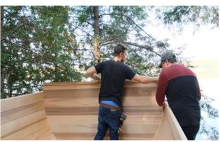
Place the window support piece onto the back wall.
