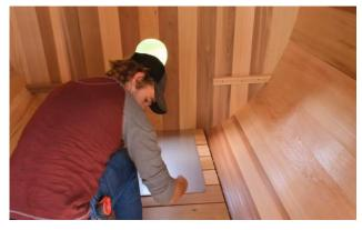
Install floor heat shield against back wall centered between the benches.
