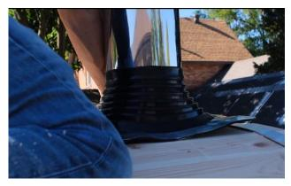
On the top of the sauna, pull the boot over the pipe, mark the outline of the boot.
