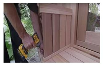
Fasten bench to floor and sauna wall using 3 - 2 ½" (64mm) screws on the top and bottom.
