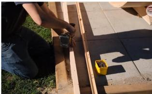
With the top stave in 2 pieces secure the spacer stave to the half of the top stave without the screws with 2" (51mm) screws.
