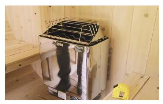
Hang the heater on the 2 screws and tighten to secure stove in position.
