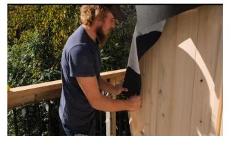
Fold the ice & water shield over the front of the staves.
