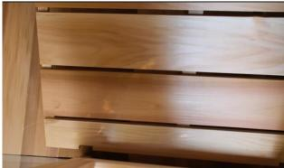
Place the flat floor so the notches are aligned with the door frame.
