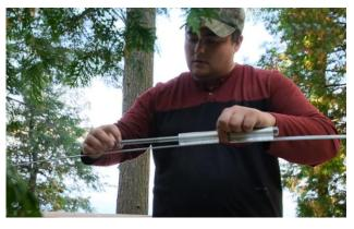
Pre-assemble the front and back bands and thread the nut on just enough to hold it together.
