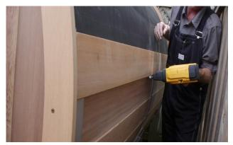
Fasten the bevel siding to the sauna using a staple gun with 1 ¼" (32mm) crown staples.
