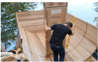
Place the door panel into the front groove of the sauna and ensure it is level.
