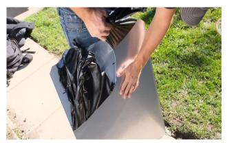
Remove all protective film from stainless steel parts and the plastic wrap from stove pipe pieces before installation.
