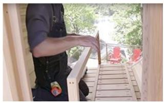
Using the pre drilled holes, assemble the lounge bench support to the longer front lower bench wall using 2" (51mm) screws.
