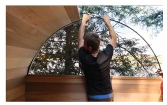
Slide the rear half moon window into the groove on the back wall and make sure it is snug into the wall.
