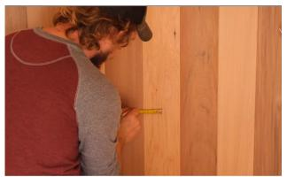
On the center of the back wall, measure 22" (56mm) from the floor up.
