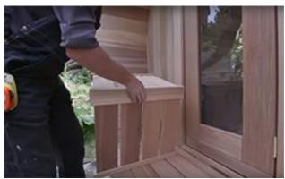
Assemble the seat and front enclosure together using 2 ½" (64mm) screws.
