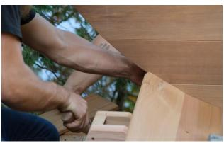
Secure every 2<sup>nd</sup> stave on the bottom of the sauna with the provided nails to hold staves in place. (*If required*)
