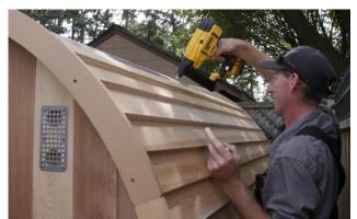
Continue adding the bevel siding using the spacer block working your way up the sauna.
