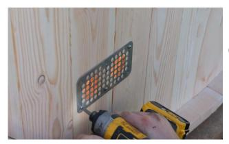
Using 1 ½" (38mm) screws, screw on the vent cover.
