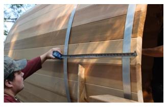
Place this band directly over the front wall panel making sure it is even all the way around the sauna.
