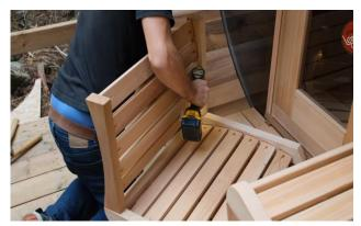
Flip the porch seat upside down and secure the front porch enclosure to the seat ensuring the contour is facing the right way using 2 ½" (64mm) screws in the pre drilled holes.
