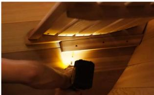
Using 2 – 2 ½" (64mm) screws per support, secure the supports to the bench seat from underneath.
