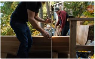
Place the provided wall support piece onto the front of the sauna.
