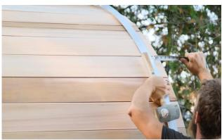
Ensure the band is 2" (51mm) from the edge of the sauna all the way around.
