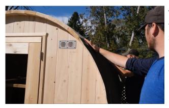
To start the installation of your bevel siding, unpeel the ice & water shield and stick it to the side of the sauna starting at the middle on one side.
