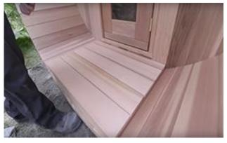
If the porch option is selected, start by installing the floor ensuring it is level.
