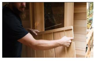
Flip the flat floor back over and it is ready to be installed inside the sauna.
