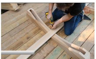
Place the center cradle centered between the front and back cradles and even on both sides of the stave.
