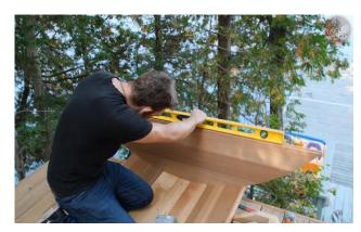
Place the back bottom wall panel centered into the groove at the rear of the sauna and ensure it is level.
