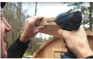
Fasten each cove piece to the next through the pre drilled holes on the front of each piece using a 2  $\frac{1}{2}$ " (64mm) screw.
