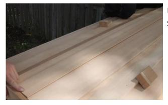
Use one last piece of the bevel siding to overlap the 2 sides.
