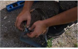
Remove the nuts and bolts from the chimney support.
