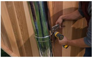
Attach a support strap around the connection and tighten up.
