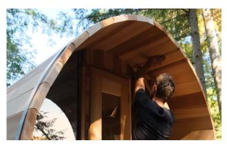
When the wall staves take on the proper shape, tighten the steel front and back bands completely.
