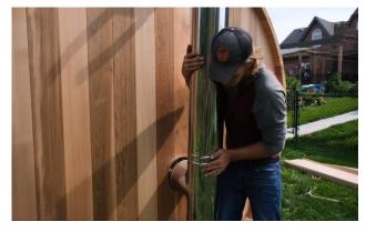
Attached assemble chimney pieces to the "T" coming out the back of the sauna.
