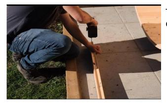
To make the top stave narrower, start by removing all of the screws from the top stave.
