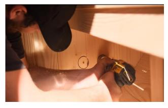
Drill out with a 2" (51mm) hole saw.
