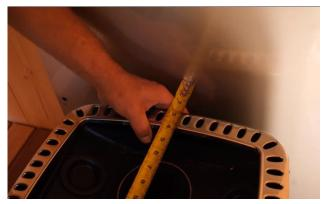
Bring in the stove and ensure it is centered between the benches with the chimney hole 8" (203mm) from the rear heat shield.
