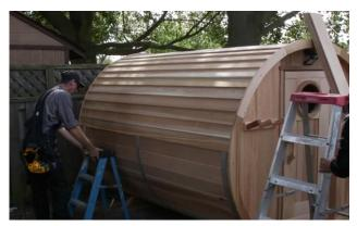
When you have installed the bevel siding up to the top, start installing the other side following the same process.
