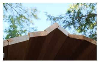
Wedge the top center stave (concave on both sides) with the last stave, to create a "V" shape.
