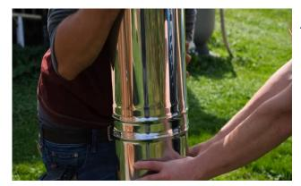
Assemble together the remaining chimney pieces.
