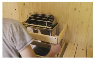
Center the guard around the heater and secure to wall with the pre placed screws.
