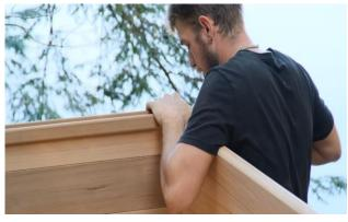
Place another stave on each side of the sauna and secure into the wall using 2 ½" (64mm) screws.
