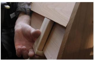
Use the provided spacing blocks as shown to get the correct placement of the next piece of bevel siding.
