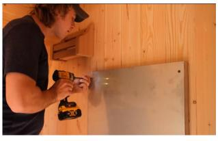
Place the rear wall heat shield and secure with 6 – 1 ½" (38mm) screws through the drilled holes.
