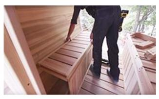
Ensure bench is flush and secure with 2 ½" (64mm) screws between the seat boards so the screws are less visible.
