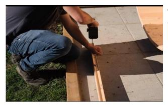
To add the spacer, start by removing all of the screws from the top stave.
