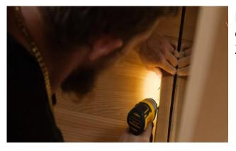
Repeat the process with the large support at the front of the sauna and secure to the wall of the sauna with  $2 - 1 \frac{1}{2}$ " (38mm) screws.
