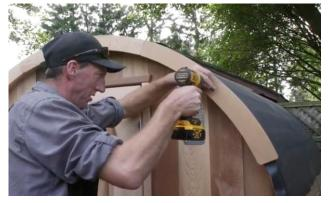
Add the next piece of trim flush to the first piece and secure with a 2" (51mm) screw.
