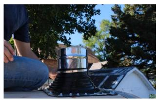
Place the hose clamp over the boot and tighten the screw.
