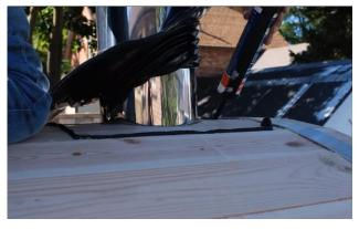
Lift the boot out of the way and apply the included roof sealer on the inside of the outline.
