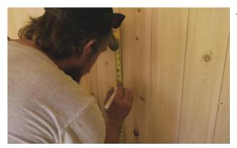
Transfer the measurements to the back wall of sauna.
