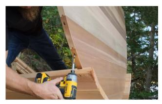
Place the middle back wall panel onto the bottom panel and secure with 2  $\frac{1}{2}$ " (64mm) screws in the predrilled holes.
