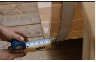
Again, ensure the front band is 2" (51mm) from the edge of the sauna all the way around.
