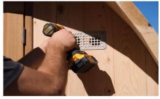
High on the front wall, repeat this process and mount the vent cover on the outside of the sauna.
