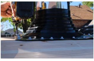
Pull the boot back down and secure with the included self sealing roofing screws 2-3" (51mm to (76mm)) apart.
