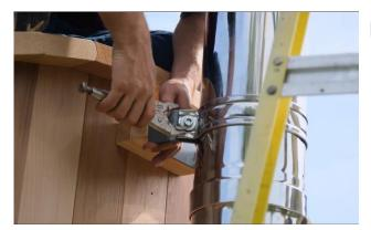
Reassemble the top chimney support bracket.
