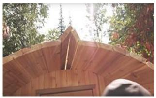
If the staves do not close together in a uniform shape, you will need to add a n include spacer
