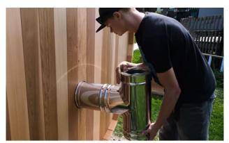
Insert the "T" chimney piece through hole in back of sauna and through the rear wall heat shield on the inside of sauna and into the back of stove.
