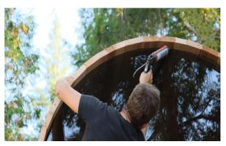
Use the caulking to seal the seams on the outside of the rear window.
