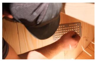
Below the bench support on the back wall, mark the vent hole position.
