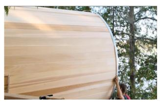
Slide the assembled band over the back end of the sauna.
