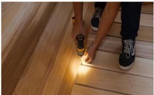
Secure with 3 - 1 ½" (38mm) screws on each side of the floor.
