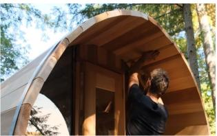
Tap out all the staves while tightening the band ensuring the staves are even.
