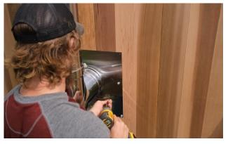
Install the bottom half of the exterior chimney shield.
