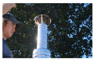
Insert the short chimney piece into the thick chimney piece, followed by the cap piece.
