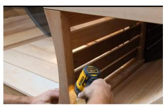
Secure to the floor and wall under the seat using 2 ½" (64mm) screws.
