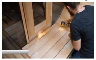
Place the porch floor with the notches for the door facing the door/
