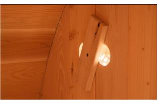
Use a 1 ½" (38mm) screw and attach the vent board on the inside of the sauna making sure it is tight but can still be turned.
