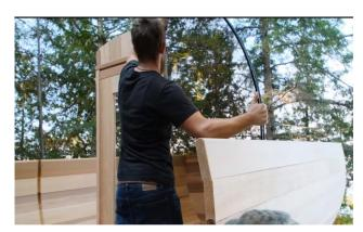
Slide the first Glass wall panel into the groove.
