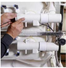
T-Type four (4) 2" drain ports allow for the drain pipe to be installed in either direction.
