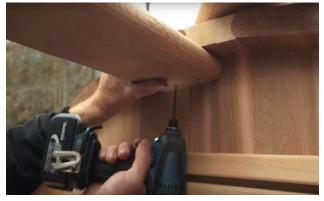
Secure with 2 ½" (64mm) screws from the underneath.
