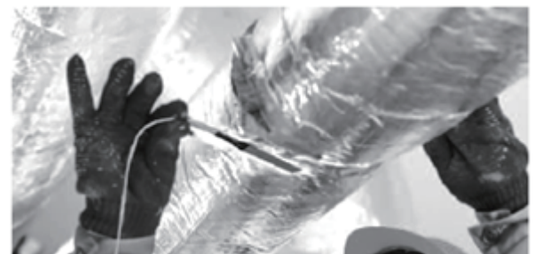
Fig. 9. Heat flow measurement of a pipe.
