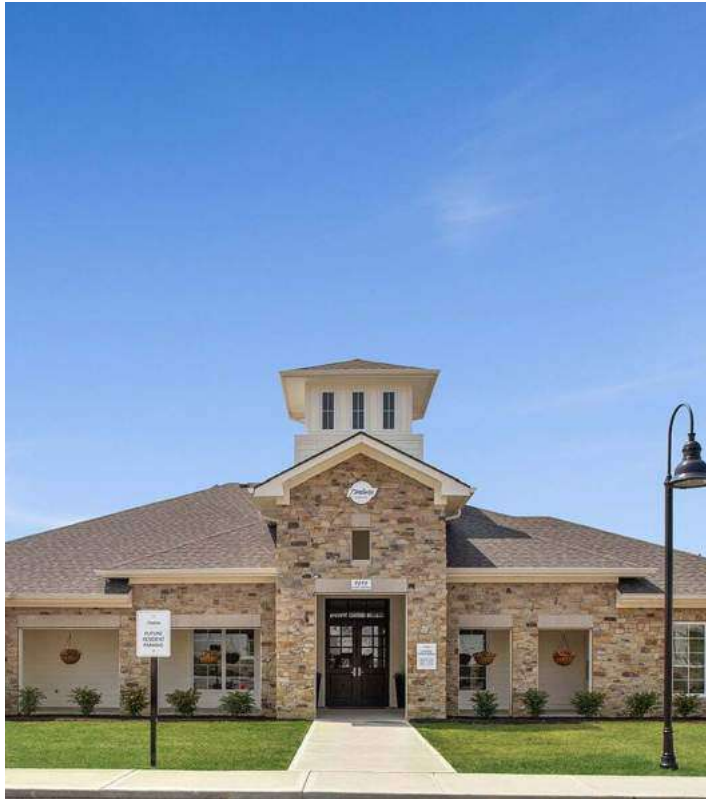
Timbers at County Line Road Indianapolis, IN
