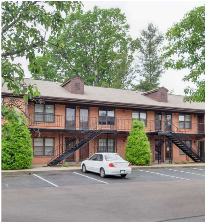
Breckenridge Apartments Louisville, KY
