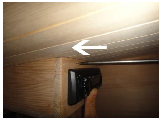
FIG 15.4 Screw wood housing to sauna room
