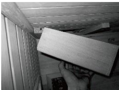
FIG 15.2 Installing the Radio Wood Housing
