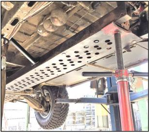
4) You will need to push the electrical lines and fuel lines slightly out of the way to make room for the top of the mid-span support. If you have the center skid plates along the underrun bars, simply unbolt the carriage bolt send it through the base of the support. If you do not have underrun skid plates, you will have to mark and drill the hole on the underrun bars before sending the included M8x80mm bolt through the mid-span support. Tighten down the Nylock nuts with the included washers.
