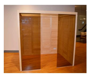
**STEP 17** - The sauna room should now have all wood and glass wall sections in place and ready for the roof installation.
