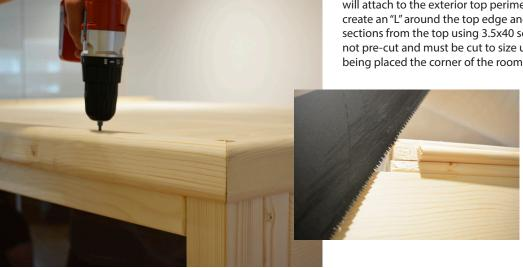
**STEP 30** - (**OPTIONAL**) Locate the exterior roof trim pieces. These will attach to the exterior top perimeter of the sauna. The pieces create an "L" around the top edge and will be screwed to the roof sections from the top using 3.5x40 screws. NOTE: The trim pieces are not pre-cut and must be cut to size using a hand saw. If the sauna is being placed the corner of the room then it is common to only install
