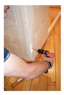
**STEP 4** - Verify that the element wall sections are square to the rails, perpendicular to each other, and that the flat top of the wall elements and corner posts align. Using a cordless drill with the appropriately sized bit (included) use 6x120 screws and secure the 90° corner post to the short and wide elements through the pre-drilled holes.
