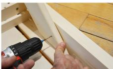
**STEP 28** - Assemble the lower bench by attaching the right and left framed leg supports to the bench and screwing into place with 4x70 screws. Be sure the two holes in the uprights are to the rear of the bench and the plastic floor protectors are down. Next, attach the angled support members so that the pins line up with the holes. We recommend to place a dab of wood glue (not included) in the holes before tapping into place. Secure the support members to the bench using 3.5x40 screws.
