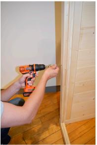
**STEP 8** - Add the third 90° corner post and secure with 6x120 screws as with the other rear corner post.
