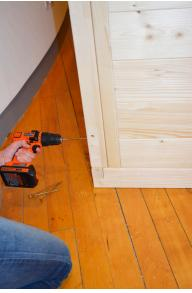
**STEP 9** - Add a wall section on the left wall and attach to the 90° corner post with 6x120 screws.
