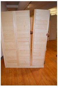
**STEP 10** - Add two more wood wall element sections along the left wall. The wall sections will not screw together, but be sure they are level at the top and firm to each other by tapping in place with a rubber mallet.
