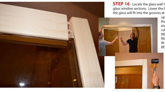
**STEP 16** - Locate the glass wall header and position over the glass window sections. Lower the header over the glass so that the glass will fit into the grooves at the base of the header. Line
