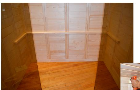
**STEP 20** - Place the upper bench onto the upper bench supports. Once the upper bench is in place, secure the rear and sides of the bench to the wall sections from below using 4x70 screws. Place one screw into each wall element section.
