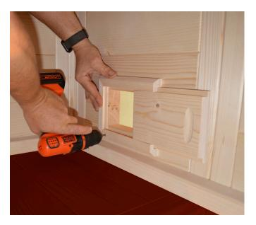
**STEP 29** - Locate the vent cover and position over the wall opening. Attach with 3.5x40 screws.
