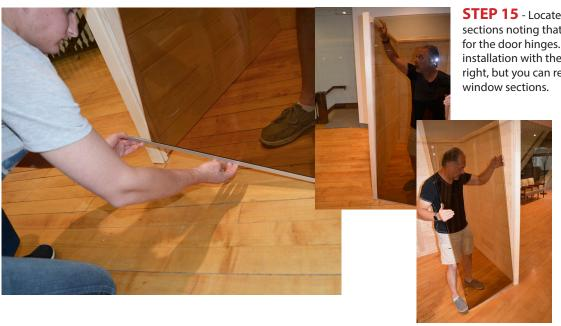
**STEP 15** - Locate the two glass window sections noting that one of them has holes for the door hinges. The instructions show installation with the door opening from left to right, but you can reverse by switching the glass
