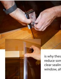
**STEP 31** - Install the hinges onto the glass door and secure to the window. The hinge consists of the hinge bracket, hole spacers, bracket cleat and hex screws. Be sure the screws are snug before mounting the door. NOTE: There is an intentional gap between the bottom of the door and the floor as well as between the glass panels. A sauna must have airflow, which
