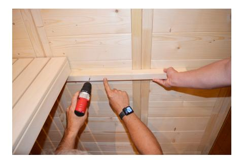
**STEP 21** - Attach the side upper bench support to the side wall by lining up to the rear side bench support. Screw into place with 5x70 screws ensuring that the support is level.
