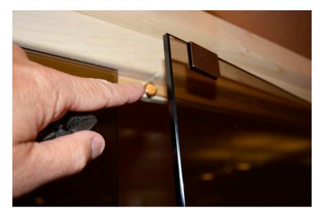
**STEP 33** - On the header above the door, peel back some of the sealing strip and find the pre-drilled hole for the magnet. Find the magnet in the hardware kit and squeeze it into the hole using pliers. The magnet is adjustable and can be loosened or tightened as needed. Cut the sealing strip to allow for the magnet and then reinsert the sealing strip in the groove.
