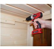
**STEP 23** - Place the upper side bench on the side bench support rail and line up to the upper rear bench. Using 5x70 screws secure the side bench to the upper bench from below. Also, fasten the side bench to the sauna wall using 4x70 screws similarly to step 20. Once the bench is securely in place adjust the metal support post by turning the black base of the post clockwise or counterclockwise as necessary to insure a solid placement on the floor.
