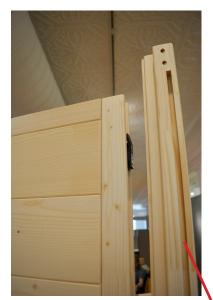
**STEP 6** - Locate one of the 90° corner posts that has clips on one side and a glass groove with 2 holes on the other. Be sure the holes are to the top and facing towards the inside of the sauna. Line up the side with the post with clips to the element section with clips. Raise the post several inches above the wall element before pushing into place. Then gently tap the post into the
