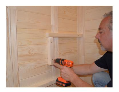
**STEP 25** - You will now install the lower bench back support. From the front of the two UPPER bench supports that you just installed, measure 1-1/2" back and make a mark. Then, install the two lower backrest supports (one on the left and right side of the sauna) to the sidewall element sections using 4x70 screws.
