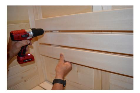
**STEP 27** - Measure 10" above the rear and side upper benches and make a pencil mark. Place one of the upper bench back supports (3-slats on each back support) above each bench and be sure it is level. Then, using 3.5x40 screws attach the back support to the wall element sections. Position your screws in the vertical battens between the slats so that the screws are concealed.
