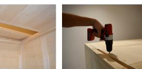
**STEP 18** - From the top of the sauna lay the (3) roof element sections in place. The side to face "up" is indicated, and the front roof section will fit into the groove of the header, and the rear roof section has a smooth edge. Once the roof sections are in place you can screw them to the roof support rails with 4x70 screws.
