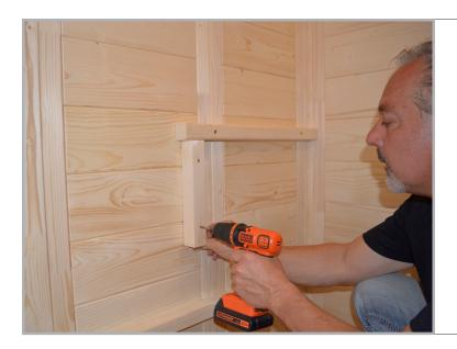
**STEP 25** - You will now install the lower bench back support. From the front of the two UPPER bench supports that you just installed, measure 1-1/2" back and make a mark. Then, install the two lower backrest supports (one on the left and right side of the sauna) to the sidewall element sections using 5x70 screws.
