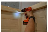
**STEP 13** - You will now install the roof support rails. Locate the (3) roof support rails and cut to length. The left and right rails should butt up to the front corner posts and the rear wall. NOTE: BE SURE THERE ARE NO GAPS BETWEEN THE WOOD WALL ELEMENTS BEFORE TAKING YOUR MEASUREMENTS.
