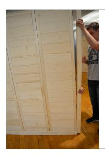
**STEP 11** - Locate the last 90° corner post that has clips on one side and a glass groove with 2 holes on the other. Be sure the holes are to the top and facing towards the inside of the sauna. Install according to the instructions in Step 6.
