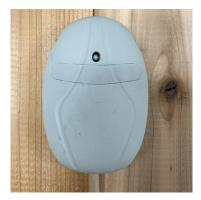
Next, feed the sensor wire out of your sauna in order to connect to the power unit.
