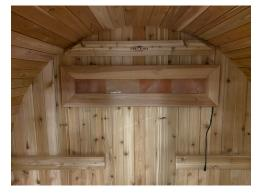
**Step 4:** Next, make a mark behind the bottom right corner of the salt bar - this will be where the power cord exits the sauna. The cord should exit behind the salt bar, and the hole should be completely covered when hung in place. Remove the salt bar and drill a  $\frac{1}{2}$ " hole completely through the wall of the sauna.
