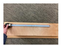
**Step 3.** Find the center point of the location you would like to mount the salt bar. 11 1/8" should be measured and marked on each side of the center point. Use a level to make sure they are at an equal height. Screw the provided installation screws at these marks, letting them protrude from the wall by approximately ½". Hang the salt bar on these screws.
