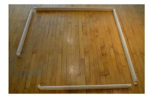
**STEP 1** - Locate the (4) bottom rails and position as shown. Overlap the corner joints and be sure the rails are square to each other. Drill a 1/8" pilot hole in the corner joints and secure rails to each other using a single 4x70 screw in each of 3 corners.
