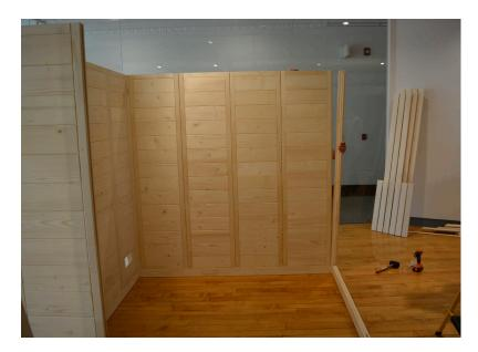
**STEP 9** - Add the third 90° corner post and secure with 6x120 screws as with the other corners posts.
