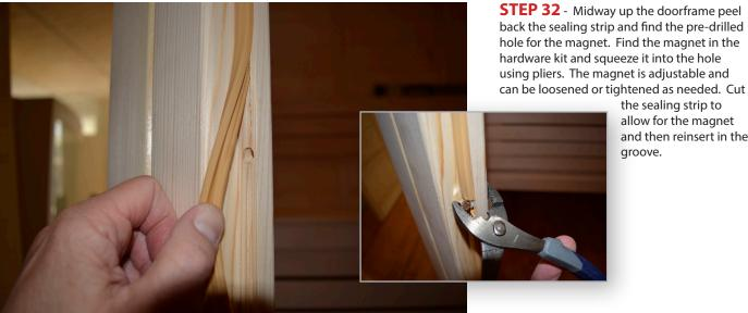
**STEP 32** - Midway up the doorframe peel back the sealing strip and find the pre-drilled hole for the magnet. Find the magnet in the hardware kit and squeeze it into the hole using pliers. The magnet is adjustable and
