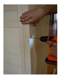
**STEP 5** - Using a cordless drill with the appropriately sized bit (included) use 6x120 screws and secure the 90° corner post to the short and wide element.
