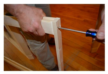
**STEP 15** - Locate the doorframe and remove the bottom board that was used to secure in shipping. SAVE THIS BOTTOM BOARD.
