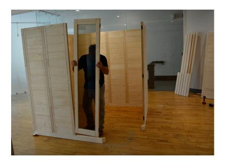
**STEP 12** - Install the narrow glass wall element section with the edge clips facing the door opening.
