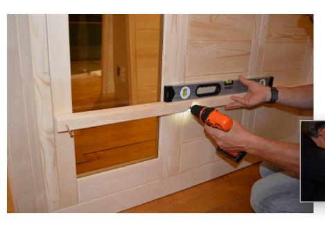
**STEP 20** - For the lower bench supports, repeat step 19 but measure up from the floor 16" and make a mark. Install the right and left longer 52" bench supports, noting that the lower bench support on the shorter left wall will cross the window and be screwed into the window panel.
