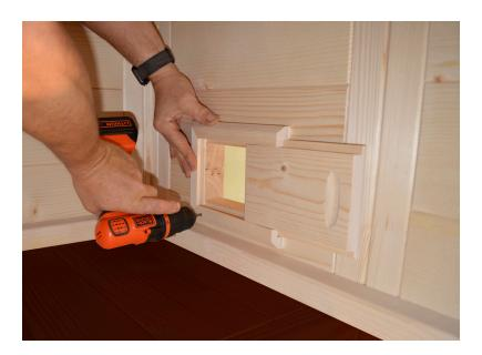
**STEP 28** - Locate the vent cover and position over the wall opening. Attach with (4) 3.5x50 screws.
