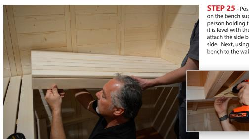
**STEP 25** - Position the side bench by placing the one end on the bench support you installed in step 24. With one person holding the bench, position the other end so that it is level with the rear upper bench. Using 5x70 screws, attach the side bench to the rear bench from the bottom side. Next, using 4x60 screws fasten the rear of the side bench to the wall element sections from below the bench.
