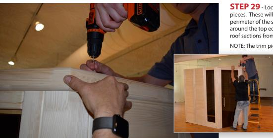
**STEP 29** - Locate the exterior roof trim pieces. These will attach to the exterior top perimeter of the sauna. The pieces create an "L" around the top edge and will be screwed to the roof sections from the top using 3.5x50 screws.
