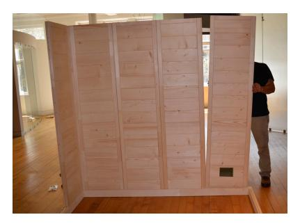
**STEP 6** - Place the next 3 wide wall element (W) sections on the rear wall, using the element with the square opening at the far right of the rear wall. There will be no screws used in these elements, but be sure the elements are firmly placed to the bottom rail and that the flat top sections are flush to each other.
