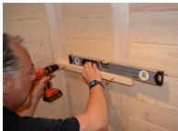
**STEP 19** - You will now install the bench supports. On the shorter left sauna wall and longer right sauna wall of the sauna, from the floor measure 34" and make a pencil mark. Position the top of the 23" upper bench support at the mark and use a level to insure that the support is level to the ground. Then screw the upper bench support into the wall element sections using 5x70 screws. Do this with both the right and left bench supports.
