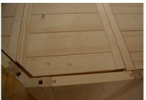
**STEP 18** - From the top of the sauna lay the (3) roof element sections in place. The side to face "up" is indicated, and the placement of the sections is intuitive. It is not necessary to screw the roof sections to the supports. A proper sauna needs airflow and should not be airtight. However, if your roof sections are not laying flat and if you can see gaps of light between the roof sections and the roof supports you can screw them down as desired to tighten the fit.
