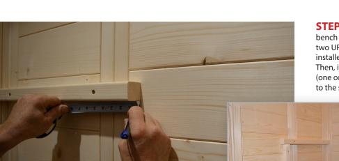
**STEP 21** - You will now install the lower bench back supports. From the front of the two UPPER bench supports that you just installed, measure ¾" back and make a mark. Then, install the two lower backrest supports (one on the left and right side of the sauna) to the sidewall element sections using 4x70 screws.
