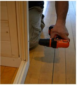
**STEP 7** - Place another 90° corner post to the end element and secure with 6x120 screws.
