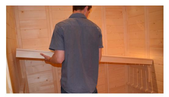
**STEP 22** - Place the upper bench onto the upper bench supports. Then, use (4) 4x70 screws and attach the rear of the bench to the rear wall from below the bench. Place one screw into each wall element section by drilling through the rear of the bench.
