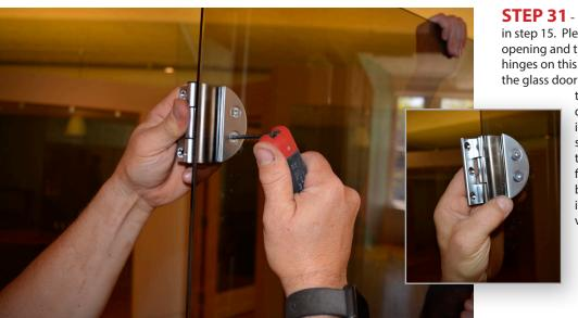
**STEP 31** - Find the board you set aside in step 15. Please it on the floor of the door opening and the place the glass door with hinges on this board. (This allows you to install the glass door with a gap at the floor) Screw
