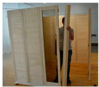
**STEP 13** - Install the (2) 45° corner posts to the narrow wall elements (one wood, the other glass) that frame the door opening. Once the corner post is in place you can nudge it into place with a rubber mallet.
