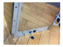
**NOTE:** While this location is the most common, the power can enter the sauna at any location. It is not recommended you use the predrilled vent holes as an entrance for the conduit.
