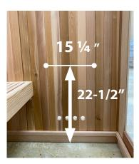
Hang the heater on the mounting screws to ensure it is level and that its base sits 5-7"off the floor of the sauna.
