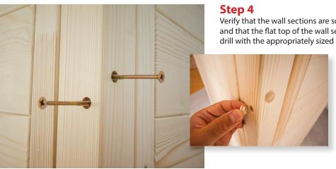
Verify that the wall sections are square to the rails, perpendicular to each other, and that the flat top of the wall sections and corner posts align. Using a cordless drill with the appropriately sized bit (included) use 6x120 screws and secure the
