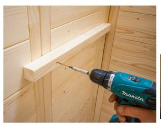
Find the two horizontal bench supports. On both the left and right sides of the sauna room, from the floor measure 32" up and make a mark. Place the bottom of the horizontal bench support at your mark and screw into place using (3) 5x70 screws each. Be sure that the bench support is level and that it butts up to the rear wall of the sauna.
