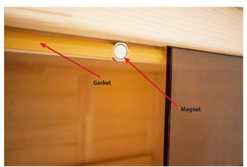
Locate the door magnet and door gasket. Insert the magnet into the pre-drilled hole above the door and push the gasket into the groove around two sides of the door (the groove that is in the door header and vertical hinge post).
