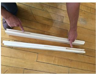
Find the door headers and select the left door header (right door header if the door is on the right.) You can determine the correct header by noting the groove for the glass window. The header will position above the door with the groove for the window to the right and facing down.
