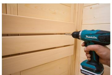
Find the back support and position the bottom 10" (+/- depending on your preference) above the bench. Using (3) 3.5x40 screws, attach to the rear wall through the vertical boards and between the horizontal slats on the rear of the back support as shown.
