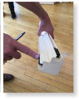
Place the 23" wall section on the front of the sauna. Using 2 people, take the 90° corner post with black plastic clips on both sides and attached to the two wall sections. Raise the post several inches above the wall sections and position so the groove and the tongue pieces align. Then, gently tap the post down with a rubber mallet so that the clips nest into each other.
