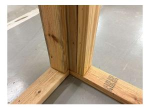
If T&G will be installed vertically, 2X4 blocking is required between the studs. Blocking is required at the base, top, and at least every 16" in between.
