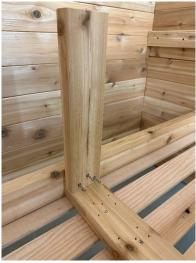
Repeat this process for the front vertical brace on the lower bench. Once the lower bench is done, repeat for the upper bench. Instead of measuring to the floor, measure from the top of the lower bench to the 2X4 brace for the front brace. For the rear brace, one is provided to follow the same process as for the lower bench (measuring floor up). You may also screw through the rear 2X4 brace into the wall, this will provide the support and vertical brace would not be required.
