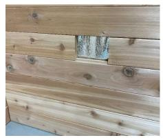
• If your heater model comes with a temperature and/or humidity sensor hardwired to the unit, find the location per manufacturer instructions. As you are installing the wall where the power unit is, we recommend drilling a hole or notching the tongue so you can route the cable out near the power unit. The cable then can easily be concealed using a cable concealer (not provided) to its location.
