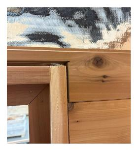
Once all the walls are installed, it's time to install the ceiling. Follow the same installation process used for the vertical walls. Unless otherwise noted, the ceiling T&G boards will run perpendicular to the ceiling joists. (Picture has some vapor barrier removed to show T&G orientation to joists.)
