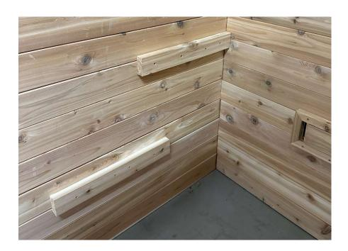
If your benches have a long span and your kit comes with vertical braces, follow the steps to install the vertical braces. This also pertains to benches that may not have a wall to fasten one end to. If your benches do not require vertical braces, skip forward to installing the benches.
