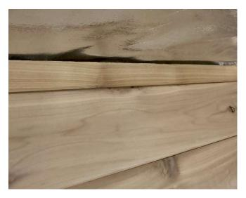
Following the same process as the side walls, install the back and front walls. Again, these T&G boards will be slightly short for ease of installation and prevent marring of side walls when positioning. Any gaps that appear in the corners will be covered by corner trim. If your door is centered and has T&G on both sides, periodically check the boards are even on both sides; you can use a full-length wall board as a guide. This will be important once you get to the top of the rough opening.
