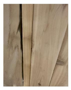
Following the same process as the first wall, continue installing the remaining walls. Again, these T&G boards will be slightly short for ease of installation. Any gaps that appear in the corners will be covered by corner trim.
