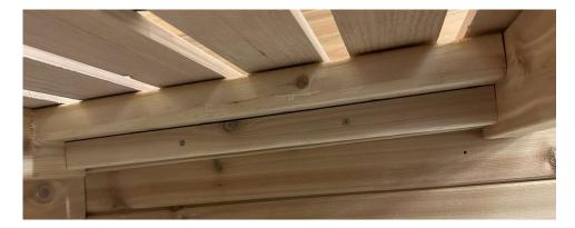
For upper benches, drill holes through the 2X4 that's against the wall every 12"-16" and fasten to the wall.
