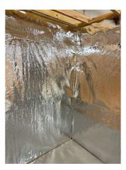
You may also choose to tape seams with foil tape (not included). Complete the same process for the ceiling as well. We recommend to have an overhang down onto the walls, so there is no gap in the barrier in the corner where the walls meet the ceiling.
