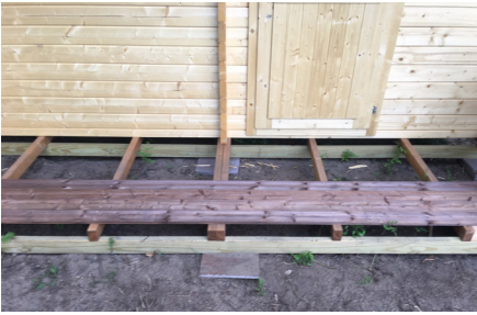
42. Install the porch (terrace) boards (TB1-1) starting at the front and working your way back toward the sauna. Place the narrow porch board (TB1-2) at the front and between the front porch rails. Nail the porch boards to the foundation stringers. NOTE: If the porch boards do not reach far enough to cover the left and right stringers, you can nail a support piece into the stringers and nail into it.
