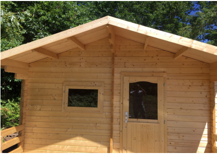
41. View of sauna after fascia boards attached.
