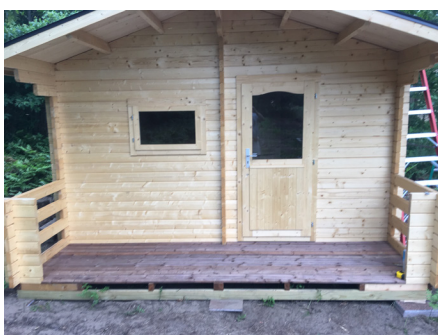
43. View of completed porch.
