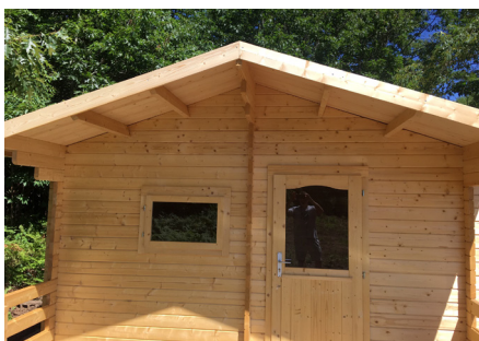
41. View of sauna after facia boards attached.
