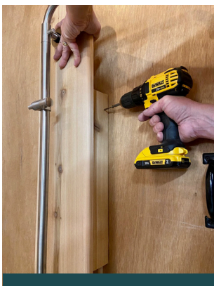
5. Screw shower mount to mounting board on both sides using 2" screws.
