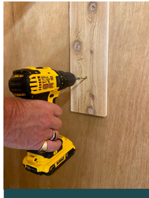
3. Screw mounting board to surface using 3" screws.
