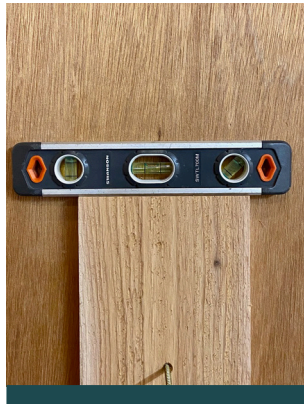
2. Check that mounting board is level and perpendicular to ground or floor.
