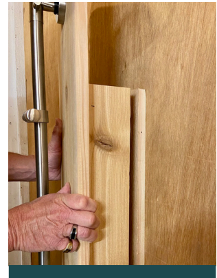
4. Fit shower mount over mounting board as shown.
