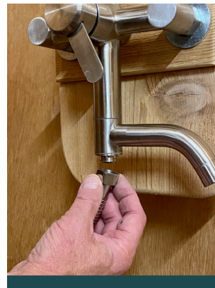
7. Attach hand wand hose to shower fixture as shown.
