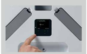
In three steps, the integrated commissioning wizard assists you in setting up the ventilation system exactly as required. The commissioning process concludes with an automatic system test and confirmation. This allows you to put the new comfort ventilation unit into operation easily, quickly and safely.
