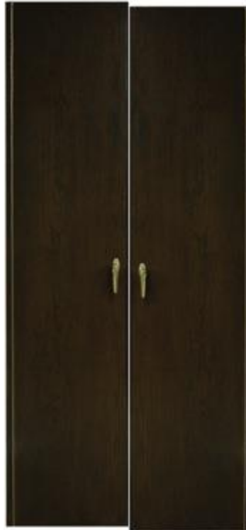
DOORS UNALIGNED: LEFT DOOR IS HIGHER THAN THE RIGHT
