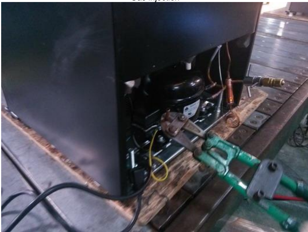
Nip the process tube (gas injection tube)
