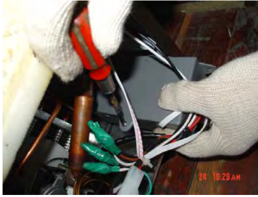
6-1-11、 Put on the control board cover.
