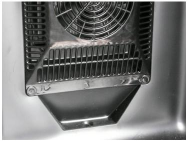
d. If ice has accumulated on the fan cover, try turning the cooler off until the ice melts away.
