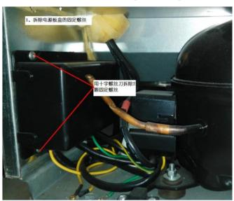
2. Remove the power board box lightly by hand.
