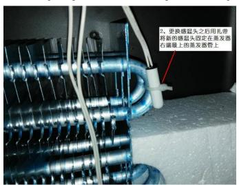
(3) Wrap up the fixed sensor of defrosting with the aluminum foil tape.
