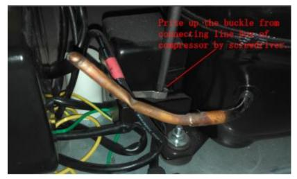
2. Remove the connecting line box slightly pressing by hand.
