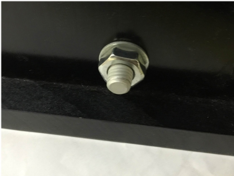
Peg Installed (Rear)
