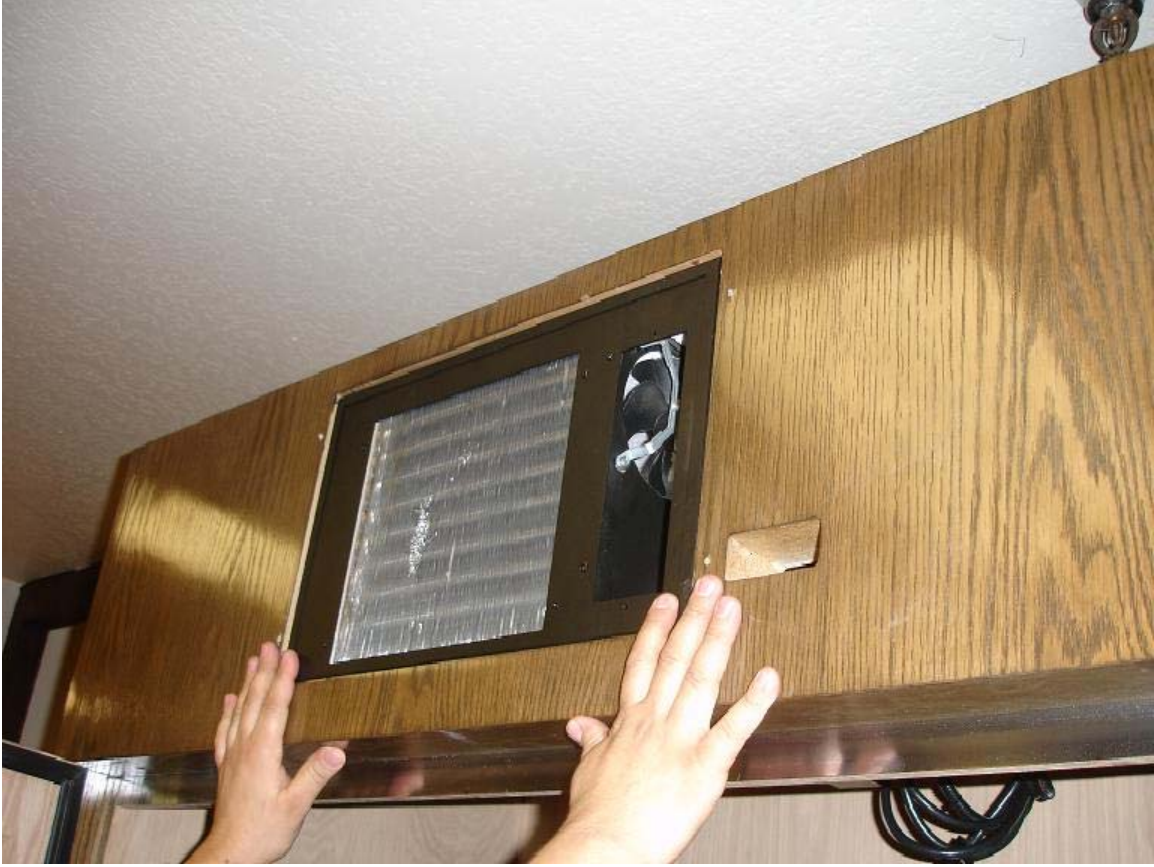
Step 2: Slide cooling unit back until frame of unit is flush with cabinet's front exterior.
