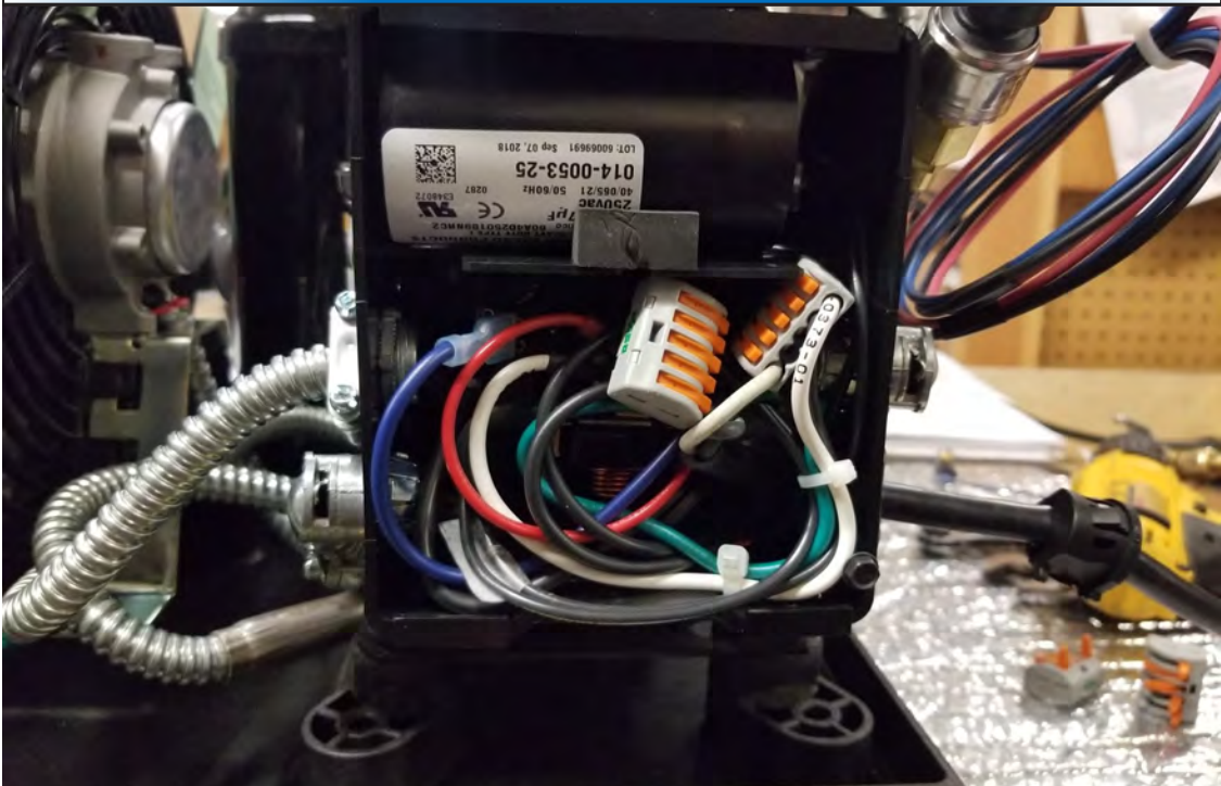
Push wires back into enclosure.
