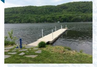
The piling anchoring method is one of the most common and popular approaches. They provide unmatched stability to the floating dock they hold; they are often the preferred option if the environment and conditions will allow for it. The anchoring of a floating dock with pilings will require the below conditions:
