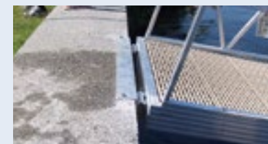
DEPARTURE ANGLE ENABLES A GANGWAY TO BE ATTACHED TO A STRUCTURE.
