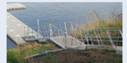
HANDRAIL INCREASES THE GANGWAY'S RIGIDITY AND SAFETY.
