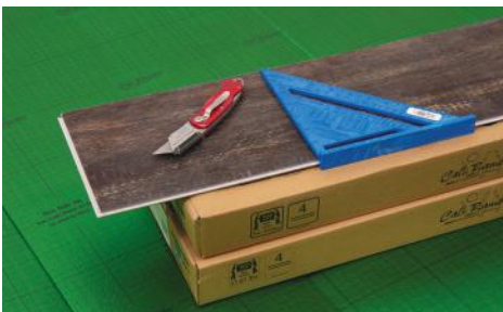
Cutting boards using Score and Snap technique
