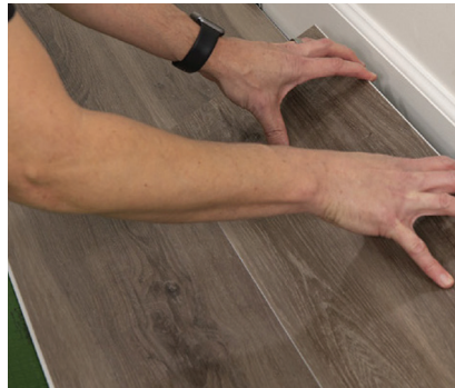
Diagram A For now three onwards, installation does not require alternating rows.
