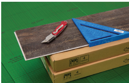
Cutting boards using Score and Snap technique
