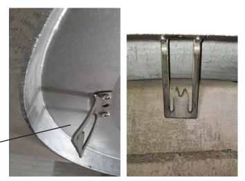
Bend the steel prongs out so the top ring is a tight push fit into the concrete capping.
