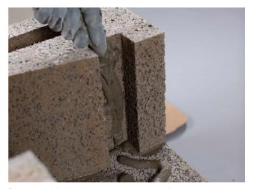
Press one side block into place and apply lip glue into the slot as shown.
