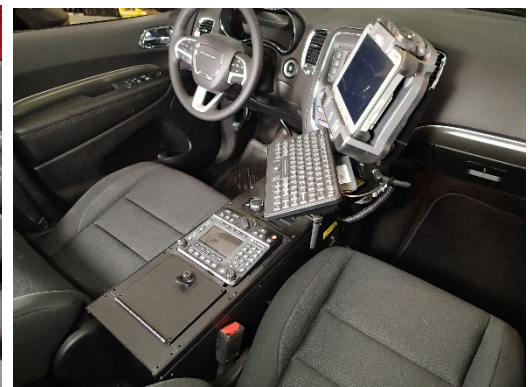
Installation is now complete
