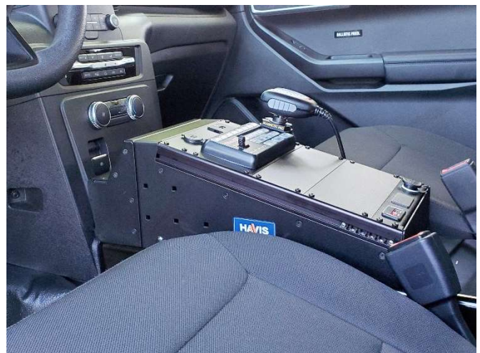
Wire and install equipment as needed. Installation is now complete.
